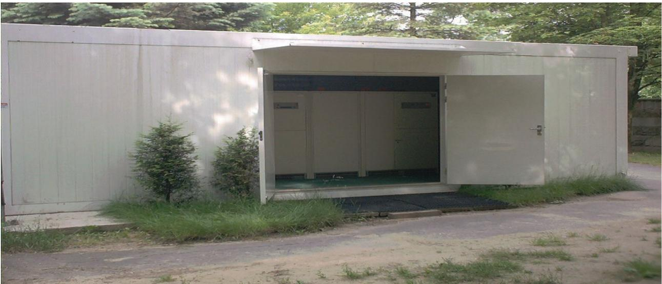
Fig. 1. A UPS container with two UPS units
