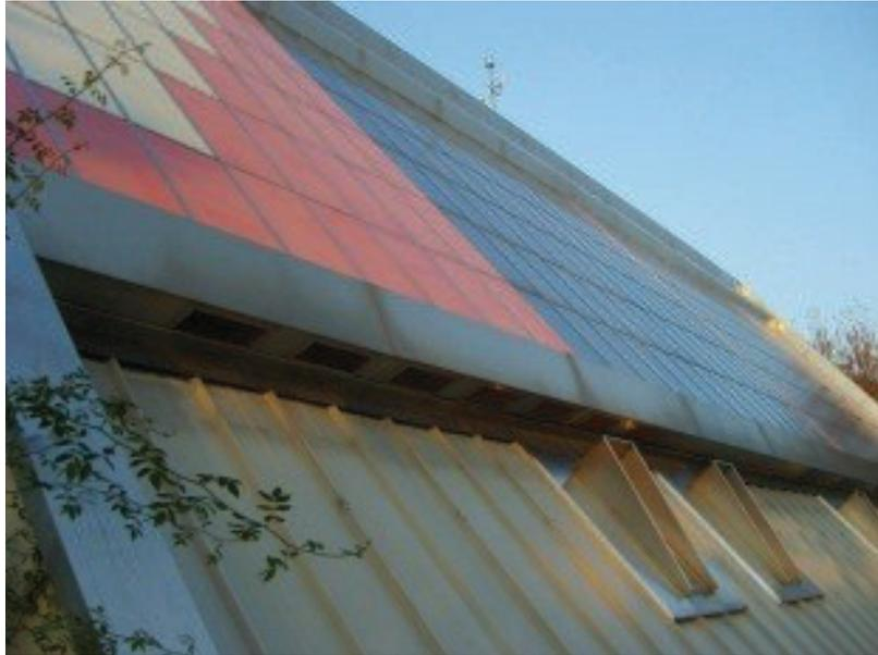
Fig. 2. The PV thermal solar hybrid façade (system) installed at the 'Eco-Canteen' of the Fiat Research Center in Turin
