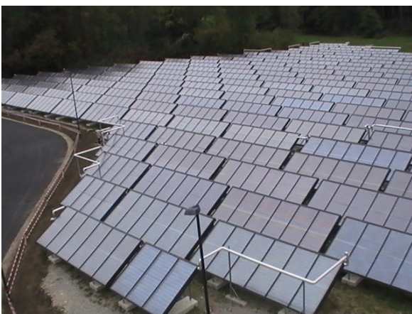
Fig. 1. An array of solar collectors of district solar heating plant in Graz, Austria
